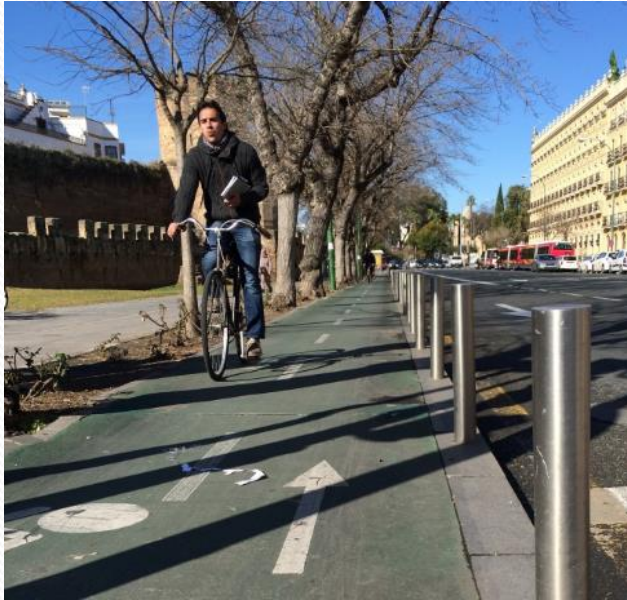
Lack of road safety Dangerous bollards (Seville)
