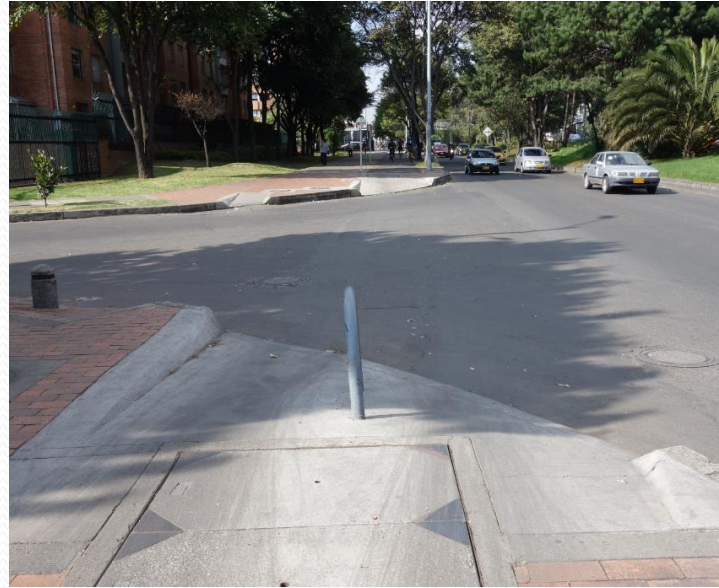
Lack of continuity / integration in traffic (Bogotá)
