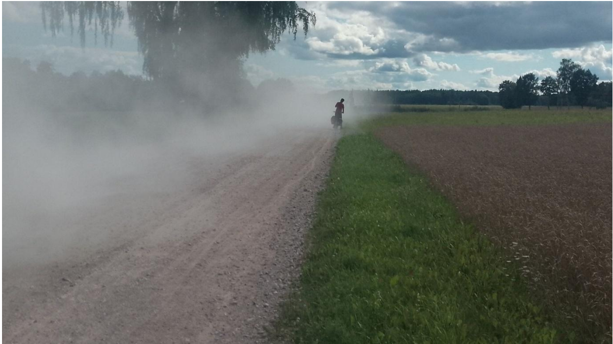
Figure 22. When exposed to sun and wind, gravel surfaces often become very dusty. Near Rokiškis, Lithuania.
