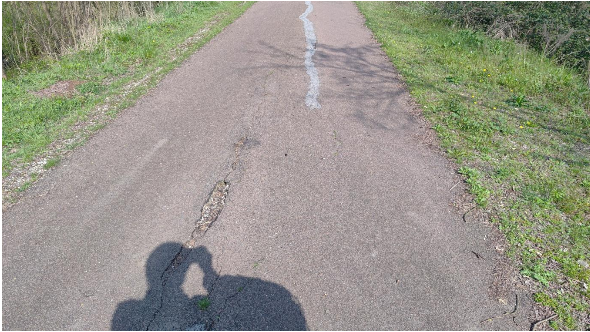
Figure 27. Triple-layer surfacing was supposed to be environmentally friendly and durable, but it is already displaying signs of age, only four years after opening. EuroVelo 7 between Osteria Nuova and Mirandola, Italy.
