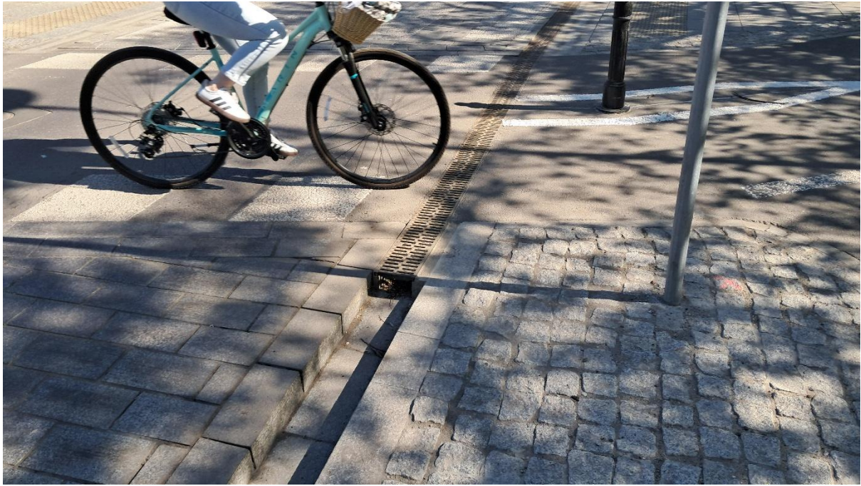
Figure 38. Gutter covered by metal grating on a raised cycle and pedestrian crossing. Andersa street, Warsaw, Poland.
