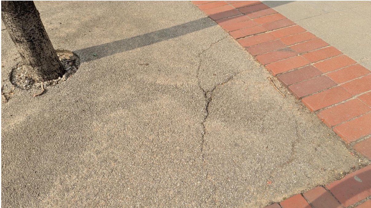
Figure 32. Resin-bound permeable surface around a tree trunk in a busy cycle and pedestrian space. Konstytucji square, Warsaw, Poland. Photo credit: Marek Smyk.
