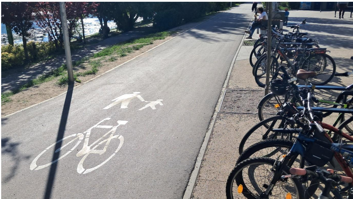
Figure 2. Different surfaces applied in an urban park setting: asphalt on the main alley (cycle and pedestrian track), concrete paving slabs on the pedestrian plaza before a cafe, resin-bound (permeable) under cycle parking and gravel with plastic structure in tree pits. Skaryszewski park, Warsaw, Poland.
