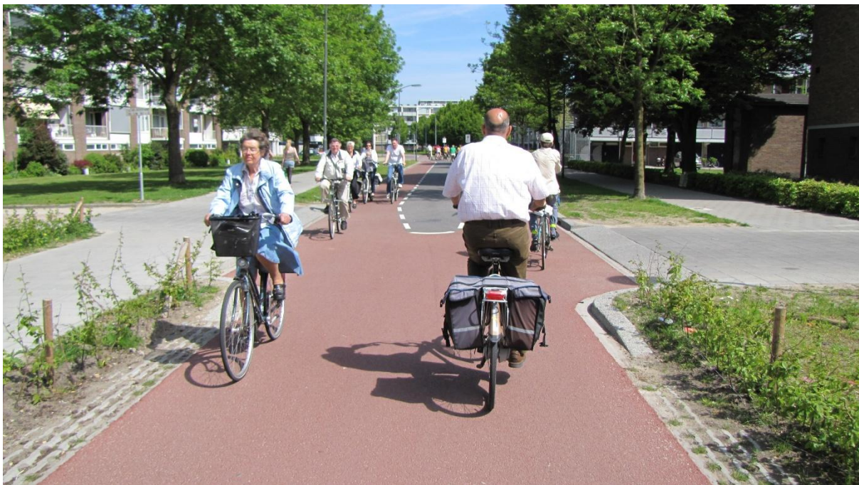
Figure 40. Consistent use of red colour for cycling infrastructure facilitates recognition of cycle routes even when the type of infrastructure changes.
