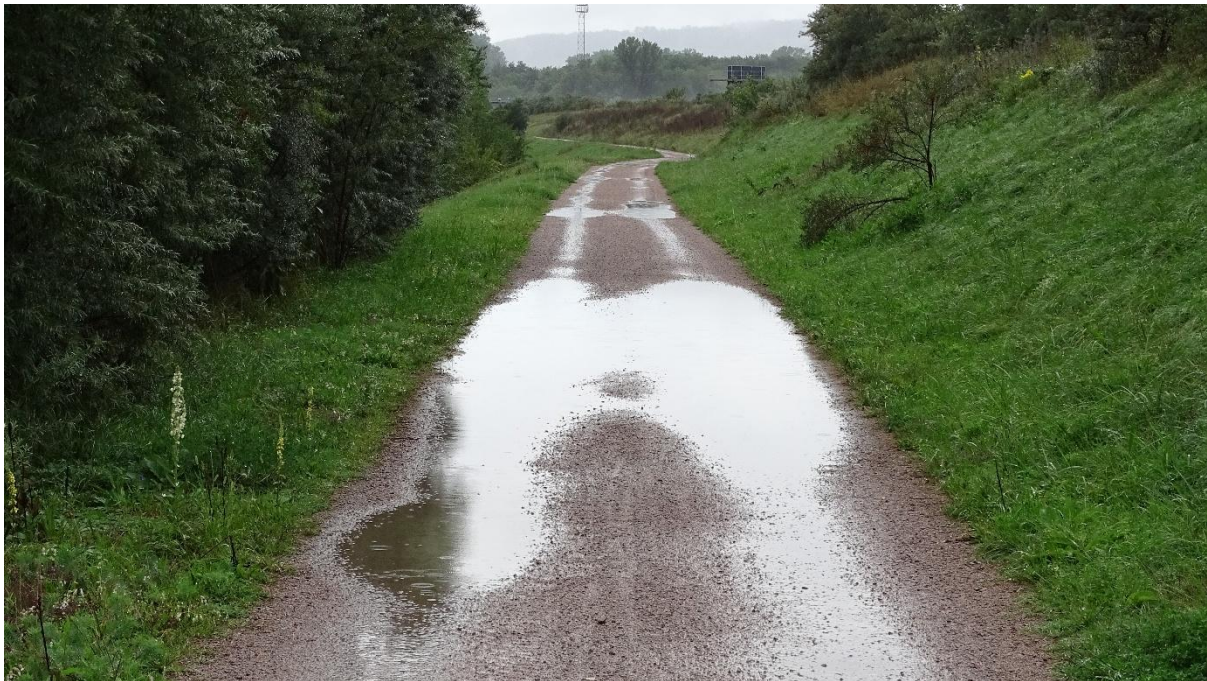
Figure 30. Contrary to a popular belief, typical gravel surfaces are generally not permeable. Near Weil am Rhein, Germany.
