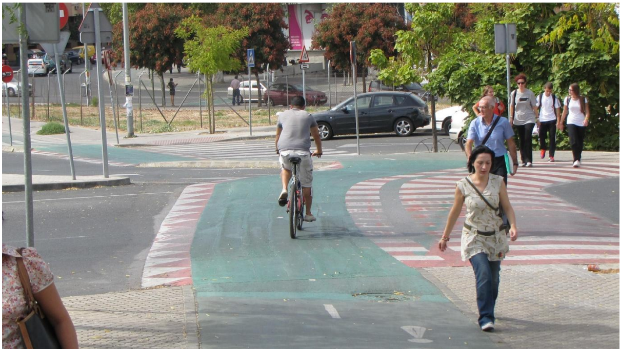
Figure 37. Continuous asphalt with no perpendicular kerb on a cycle crossing. Sevilla, Spain.
