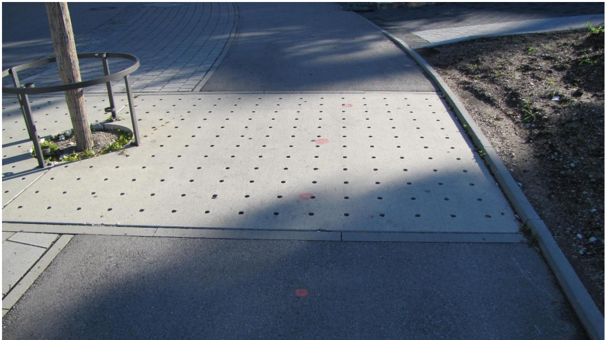
Figure 12. Concrete “bridge” over tree roots on a cycle track. Holes in the concrete plates ensure permeability for water. Munich, Germany.
