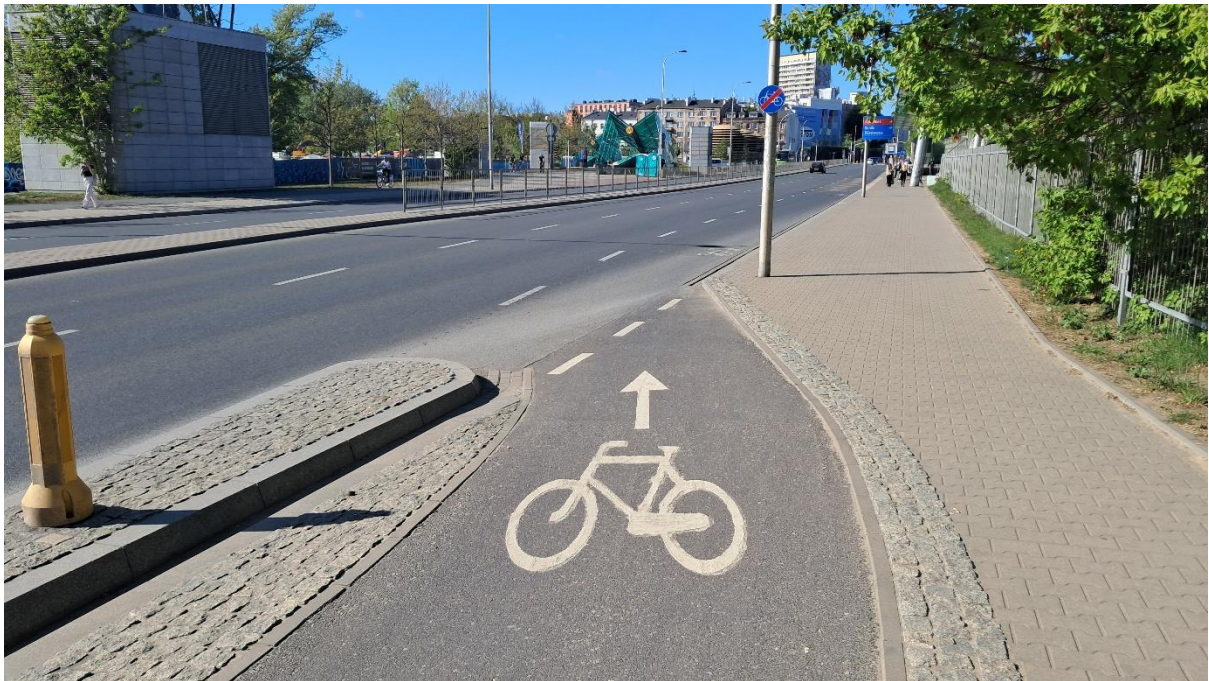
Figure 39. Gutter discontinued on the connection of cycle track and carriageway. A gutter or a kerb here would be particularly dangerous because of the angle of crossing. Sokola street, Warsaw, Poland.
