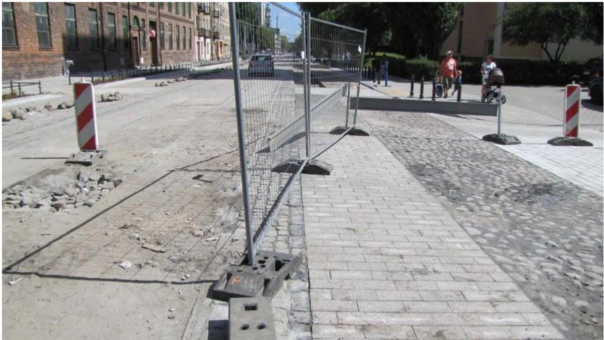
Figure 34. Clean-cut paving stones on the sidewalk and the cycle lane, cobblestones left in the parking lane and car lane. Kawęczyńska street, Warsaw.
