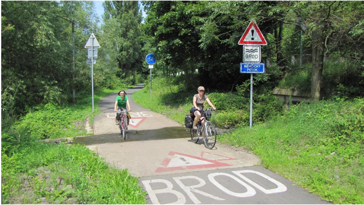
Figure 10. Concrete ford on otherwise asphalt cycle track. EuroVelo 9, Czechia.
