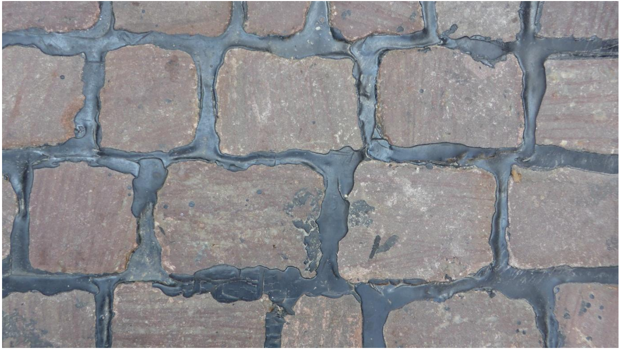
Figure 33. Clean-cut sett paving with bitumen filling between the stone blocks. Old town centre in Freiburg, Germany.
