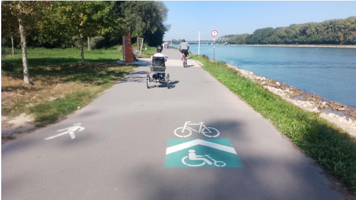
Figure 1. Smooth and even surface is one of the preconditions for accessible cycle route. EuroVelo 15 near Gemersheim, Germany.
