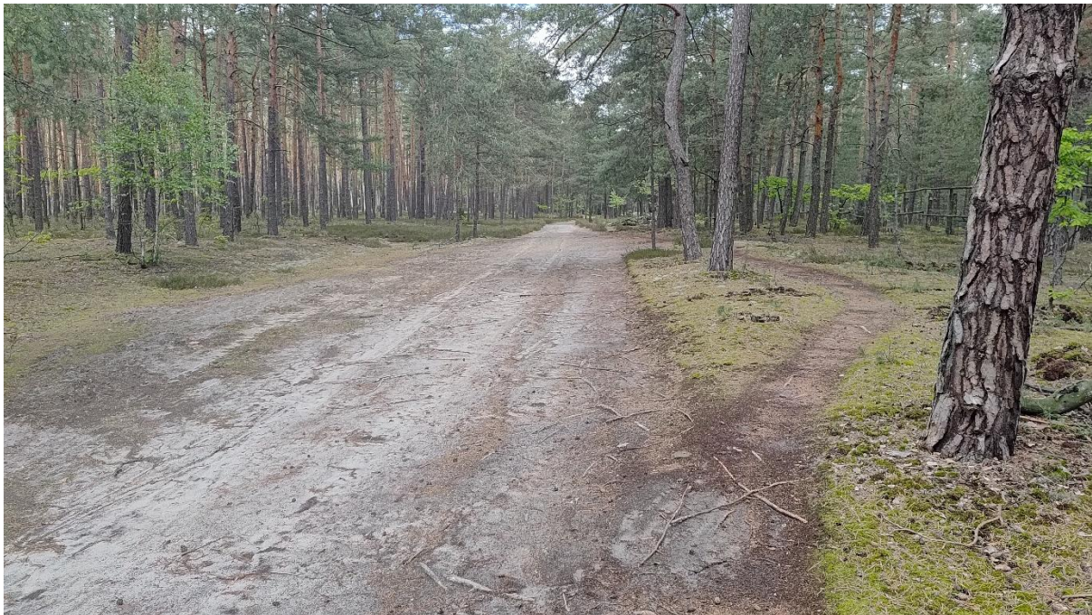
Figure 26. Unimproved surfaces become sandy or muddy with use, which prompts users to search for alternative paths to bypass the problematic area. The total footprint and trauma to local flora increases. Kampinoski National Park, Poland.
