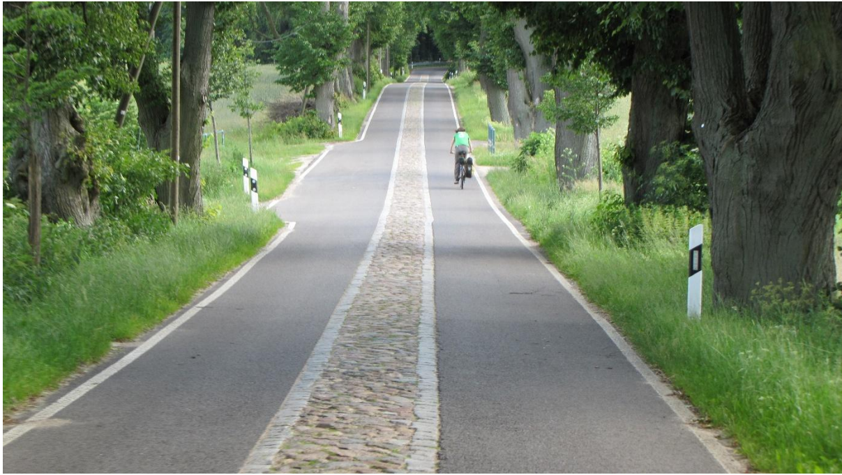
Figure 35. Historical rural alley with smooth asphalt lanes on both sides and cobblestones left in the central strip as a traffic calming element. Near Parlow, Germany.
