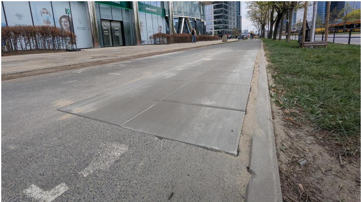
Figure 15. Paving slabs used for provisional surfacing after underground infrastructure repairs. Warsaw, Poland. Photo credit: Marek Smyk.
