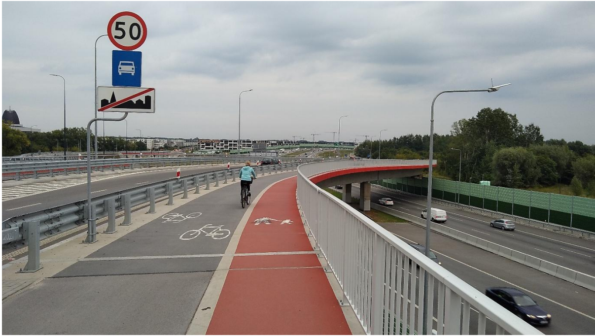
Figure 41. Around Warsaw, Poland, on network sections managed by the national road administration, red colour designates space for pedestrians. Unfortunately, the colour-coding is the exact opposite on sections managed by local municipalities (red for cyclists, grey for pedestrians).
