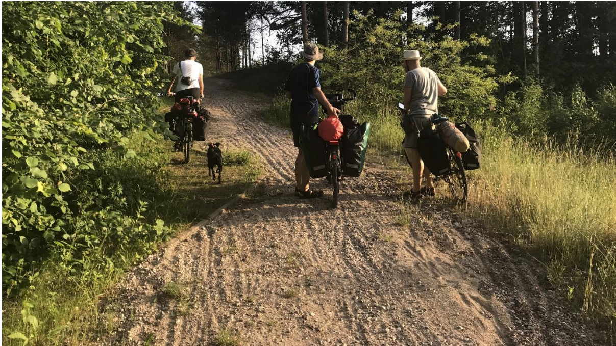
Figure 24. Deteriorated gravel surface on a slope. Green Velo cycle route, Poland. Photo credit: Wojciech Grela.
