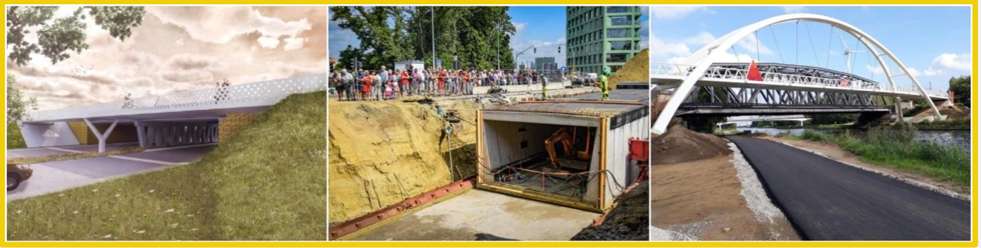
Investments planned (1), in construction (2) and ready to welcome cyclists (3)
