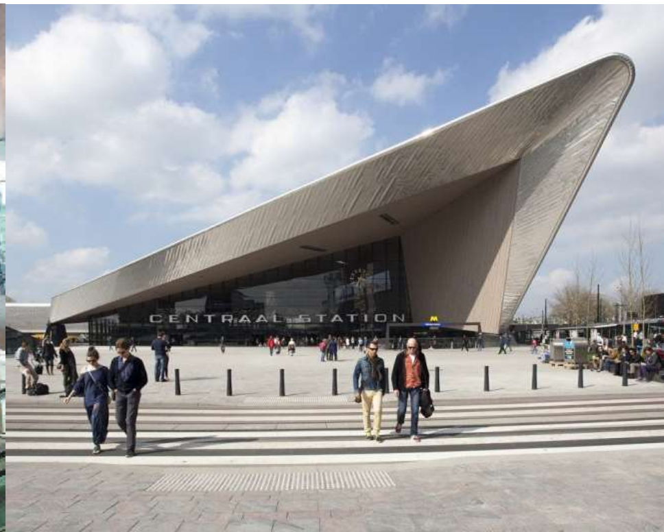
Central station in Rotterdam
